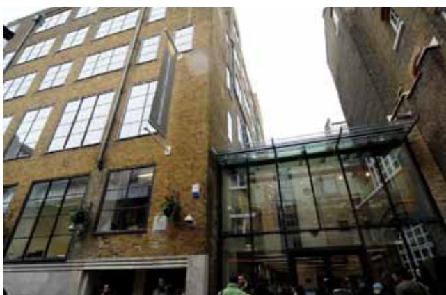
Glass entrance to IH London, Stukeley Street
